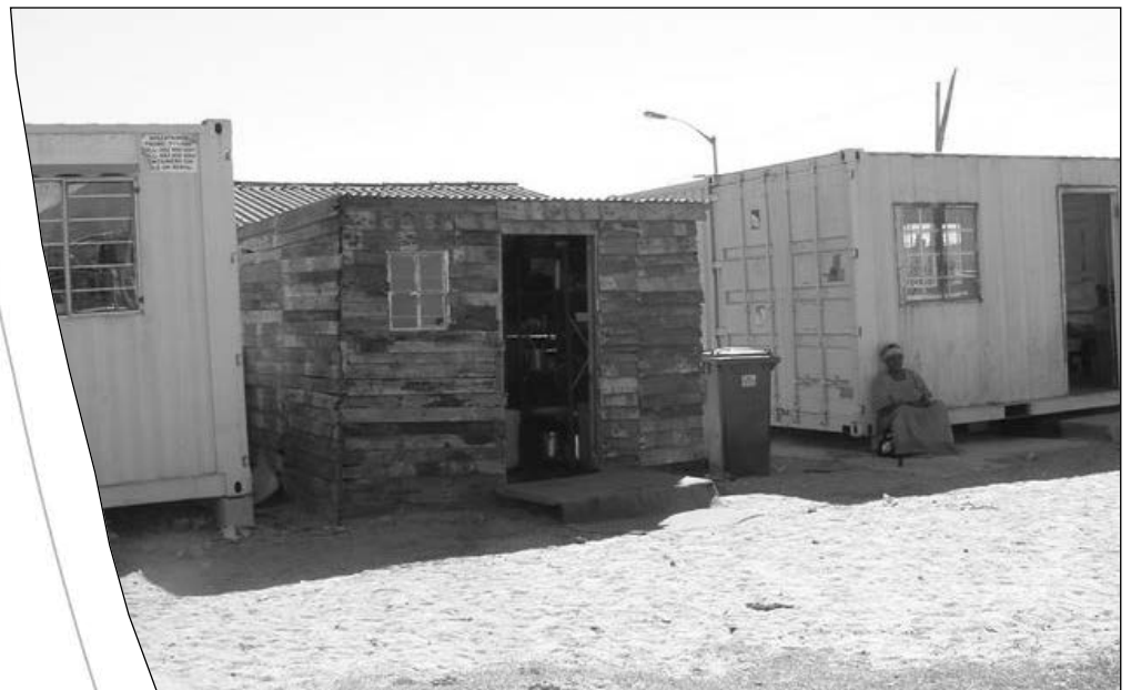
The log cabin which is the new kitchen situated between the classrooms in the shipping containers.
